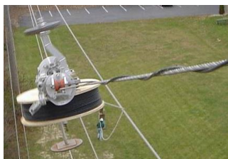
Wrapped aerial cable
