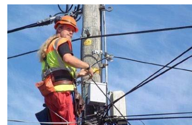
Figure 7: Aerial cable installation
