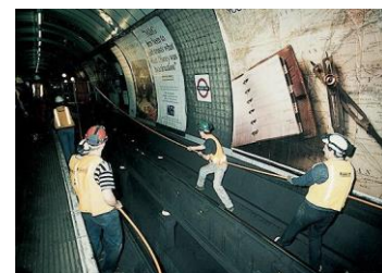
Figure 9: Cable installation in tunnels
