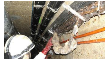
Figure 8: Cable installation in sewers
