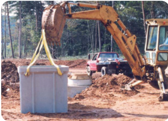
Lift and position enclosure with backhoe.
