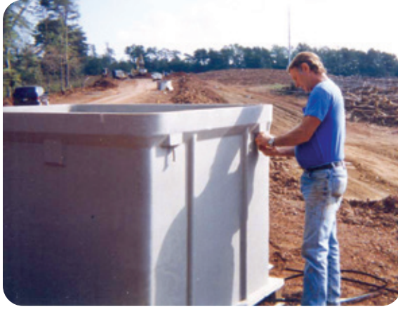
Attach nylon straps or chains to the lifting bolts.
