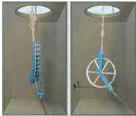
Sheaves and quadrant block in manhole
