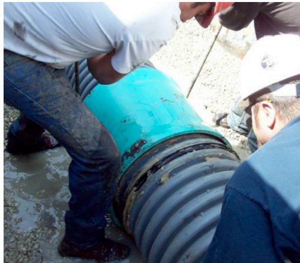
Figure 10.7: Slip Repair Coupling
