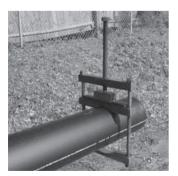
Figure 15 Mechanical Re-Rounding Clamp Installed
