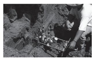
Figure 3 Saddle Fusion Repair
