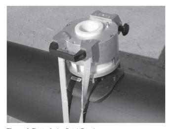
Figure 4 Electrofusion Patch Repair
