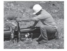
Figure 1 Above Ground Repair with Fusion Machine
