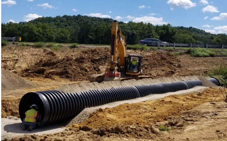
Figure 4.3: Dual-wall HDPE pipe installation
