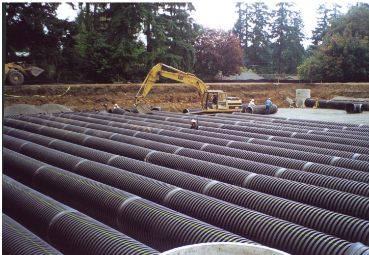
Figure 4.11: Typical detention system
