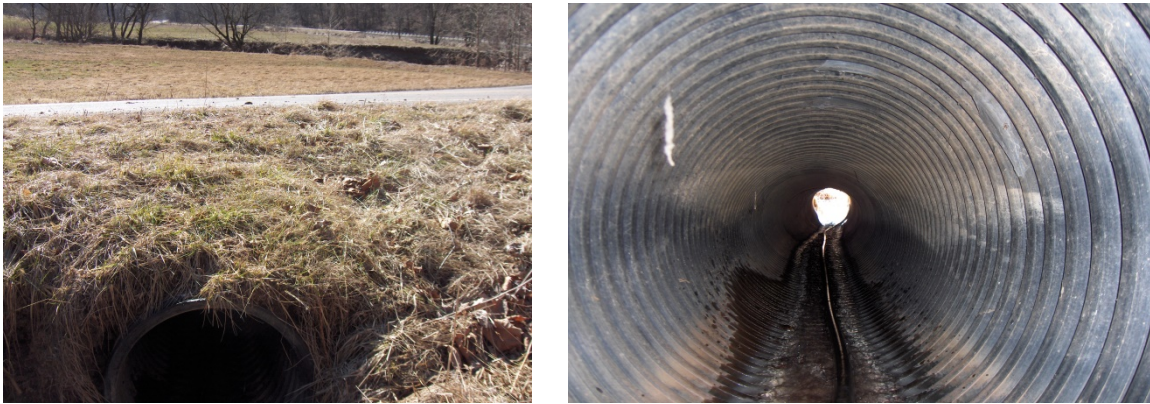
Figure 4.7: Installation of 24-inch diameter culvert since 1981 in acid mine run-off
