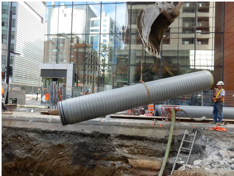
Figure 4.5: Triple wall corrugated pipe installation
