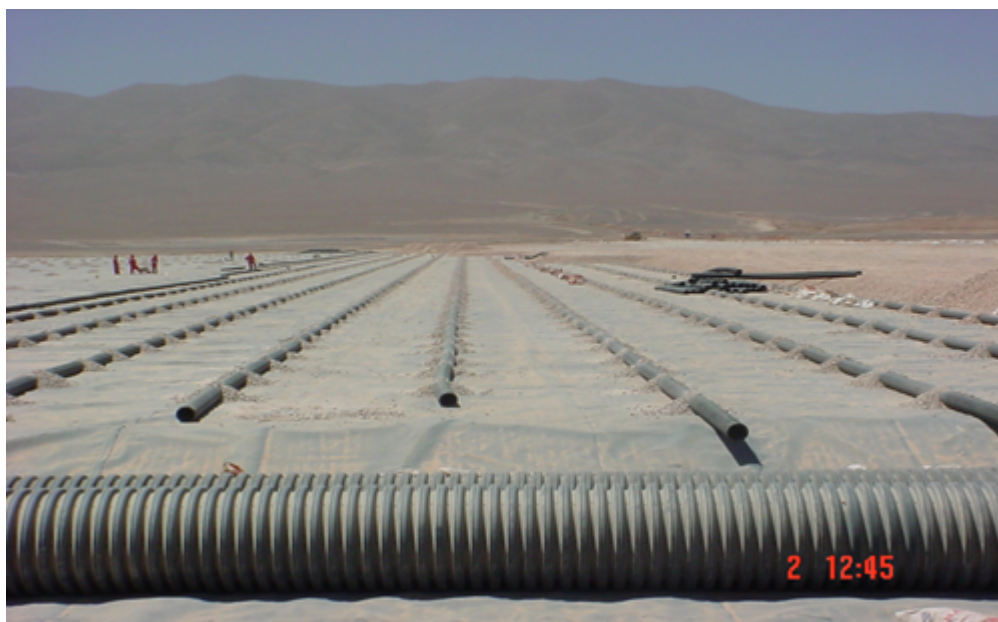
Figure 4.14: Typical heap leach pad construction
