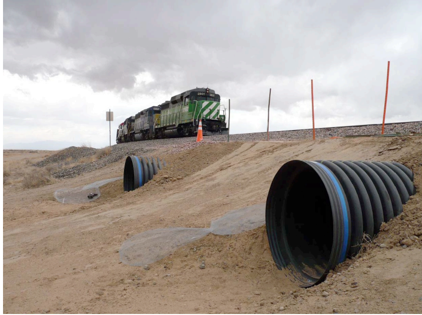
Figure 4.9: AAR TPCI test installation in progress
